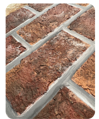
Brick work made with Dekozell
